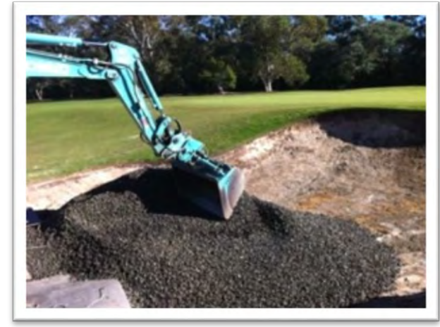
3. Spread Capillary Concrete to 2 inches depth
